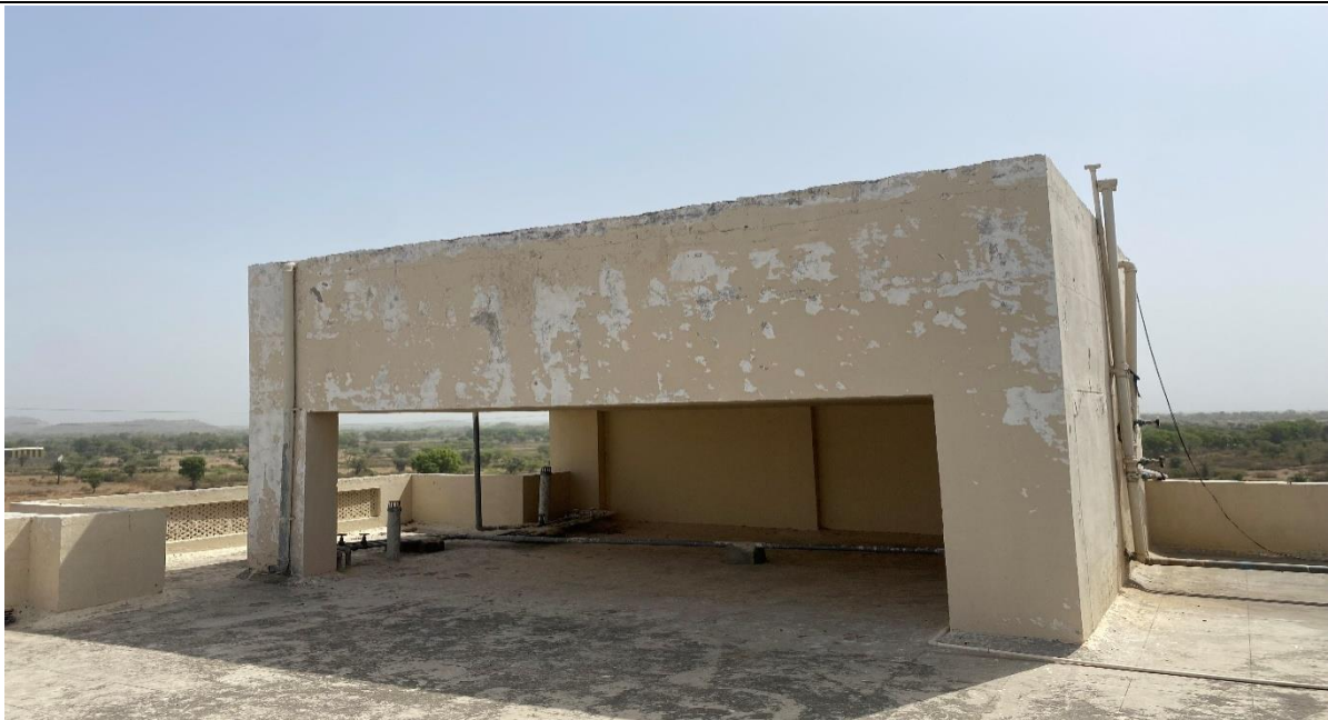
Fresh Water Storage tank
